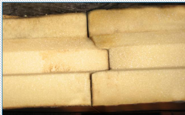
Picture 3: Insulation boards tightly installed against one another
